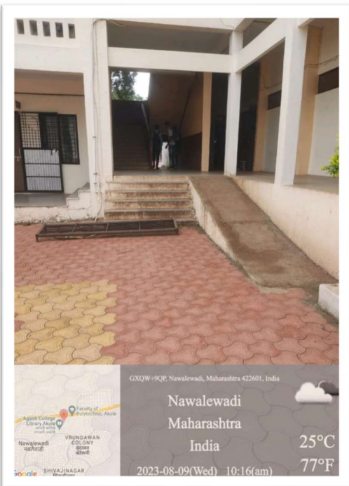
Ramp at Chemistry Department
