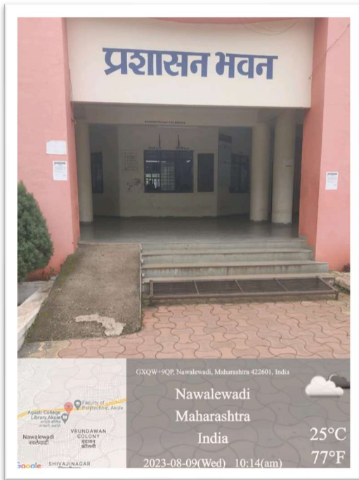
Ramp at Administration Office
